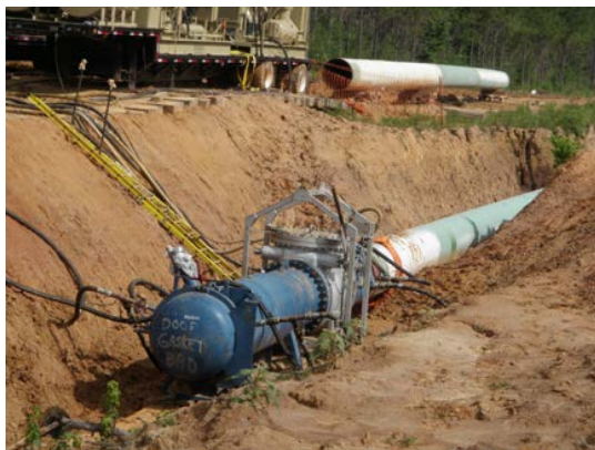
Figure 29: Drying process after hydrotest
