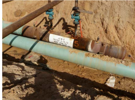
Figure 28: Hydrotest in Progress
