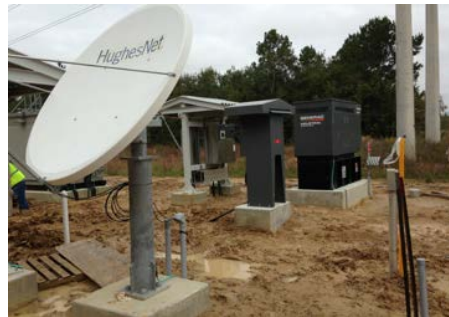
Figure 14: Remote Operation Equipment at Valve site.
