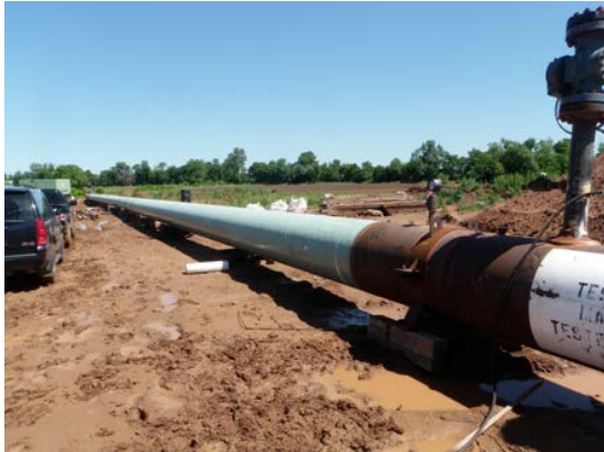
Figure 27: Hydrotest in Progress
