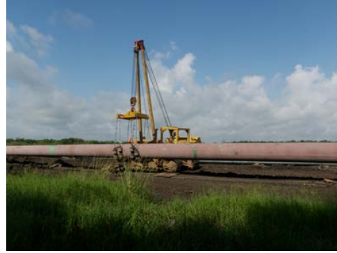
Figure 10: Boom holding Pipe
