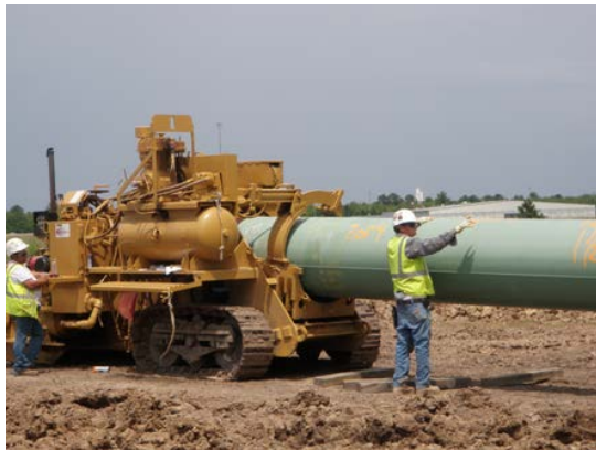
Figure 11: Bending Machine
