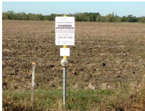
Figure 24: Typical Test Station
