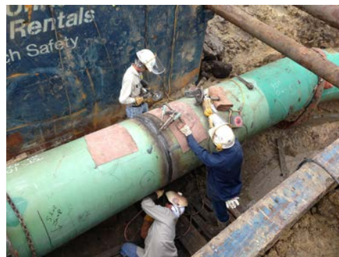
Figure 22: Manual Welding Set up
