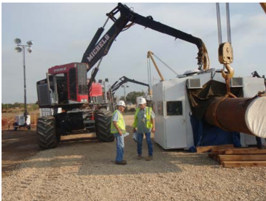
Figure 20: Automatic Welding Shack
