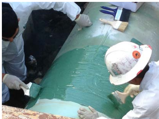
Figure 23: Coating of field joint
