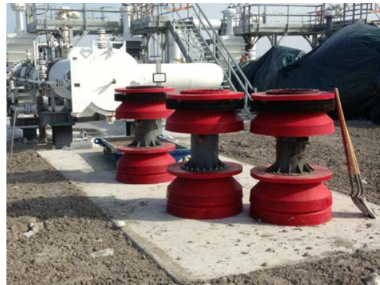
Figure 30: Pigs used during commissioning.
