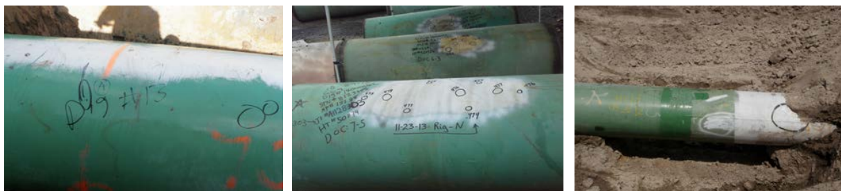
Figure 32, 33, 34 Examples of dents found with inspection tool.
