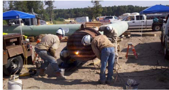
Figure 19: Welder Qualification Test
