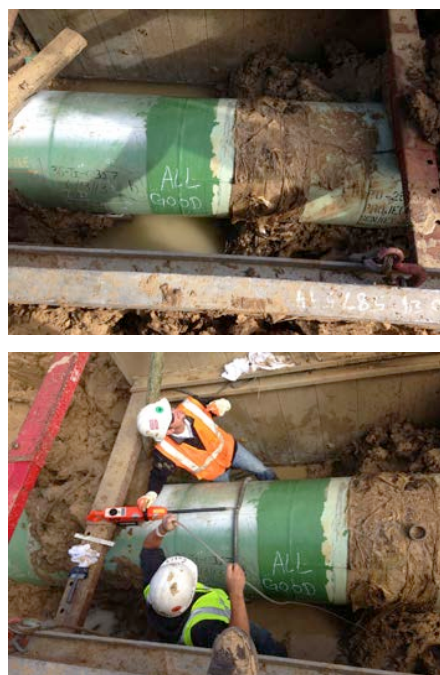
Figure 25 and 26: DCVG dig site (recoated)
