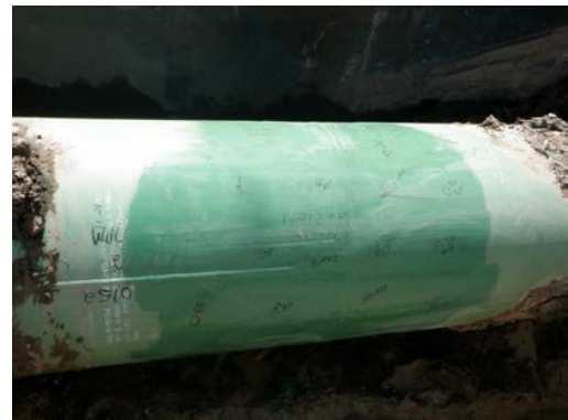
Figure 35: Repair of coating due to weld splatter.
