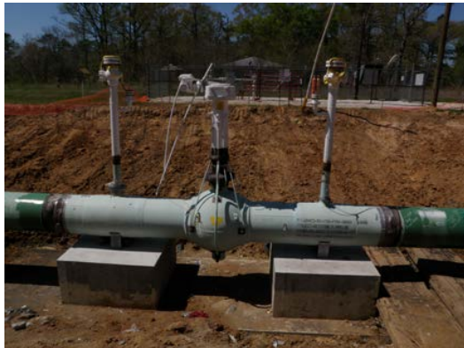
Figure 17: Concrete Pads for Valves.
