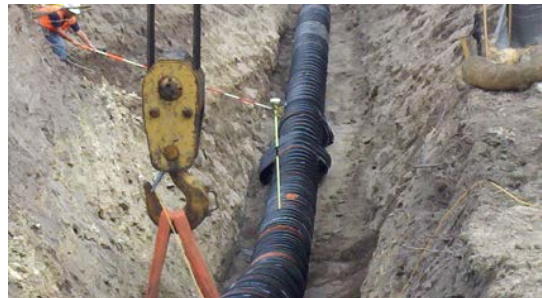
Figure 9: Depth of Cover check with GPS
