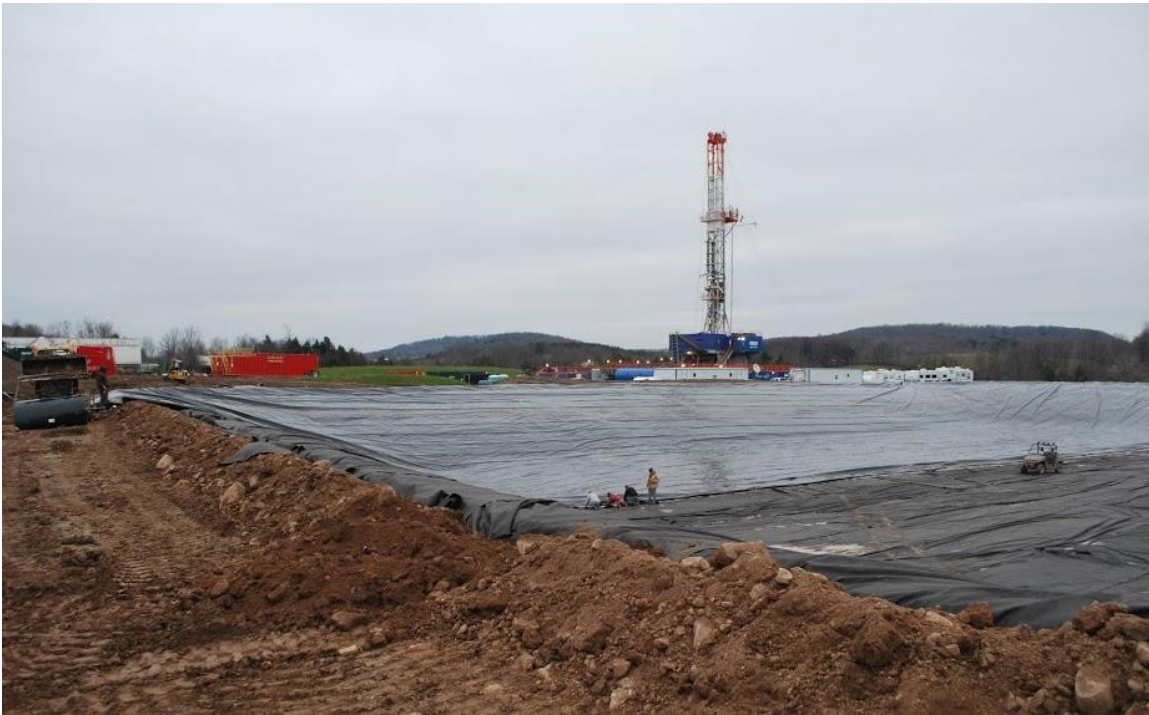
Centralized impoundment under construction in Pennsylvania. Photo by Frank Finan.
