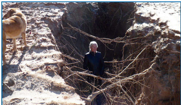
Eleanor Fairchild stands in an erosion area adjacent to a wetland after pipeline construction on her property.
