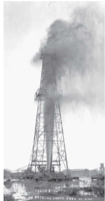
(1929) Kingsville, Texas, blowout.
