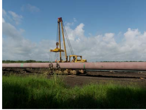
Figure 10: Boom holding Pipe
