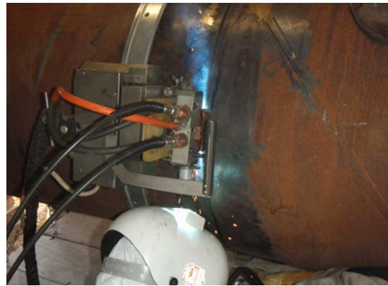
Figure 21: Automatic Welding Set up
