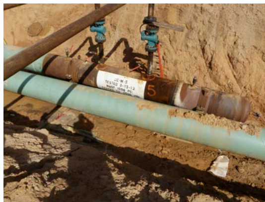
Figure 28: Hydrotest in Progress
