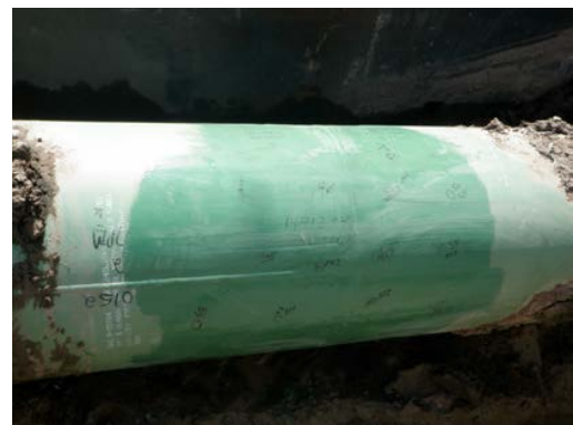
Figure 35: Repair of coating due to weld splatter.
