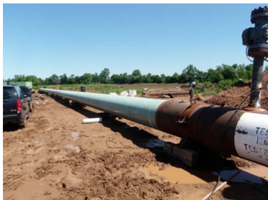
Figure 27: Hydrotest in Progress
