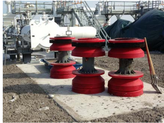
Figure 30: Pigs used during commissioning.
