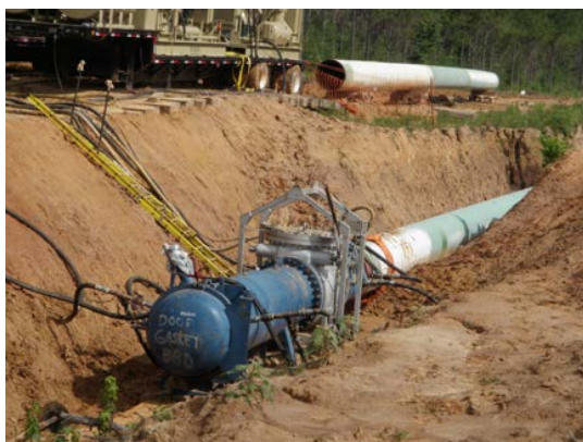
Figure 29: Drying process after hydrotest
