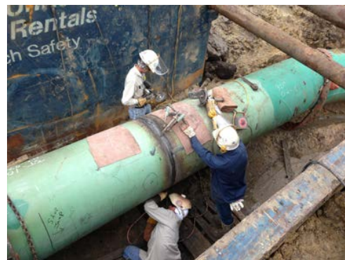
Figure 22: Manual Welding Set up
