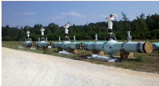
Figure 15: Valve Storage at Pipe Yard
