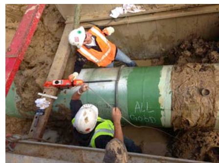
Figure 25 and 26: DCVG dig site (recoated)
