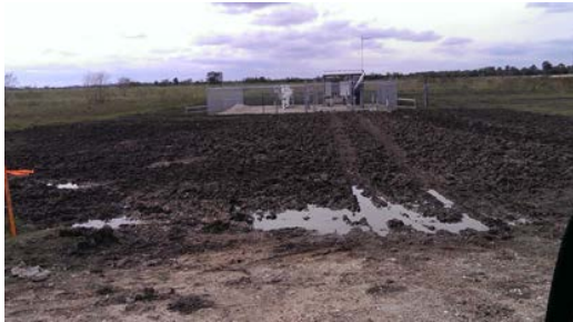
Figure 13: Typical Valve location
