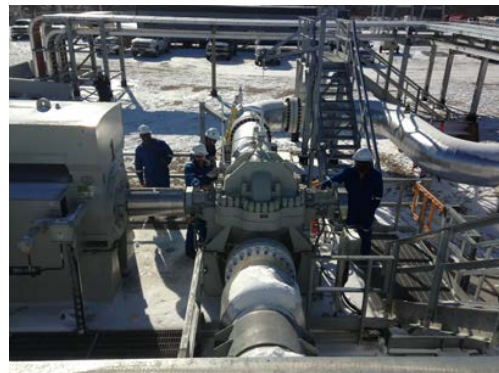
Figure 31: Commissioning at Pump Station
