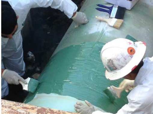
Figure 23: Coating of field joint
