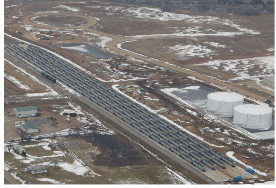
Aerial view of the Stroud Terminal
