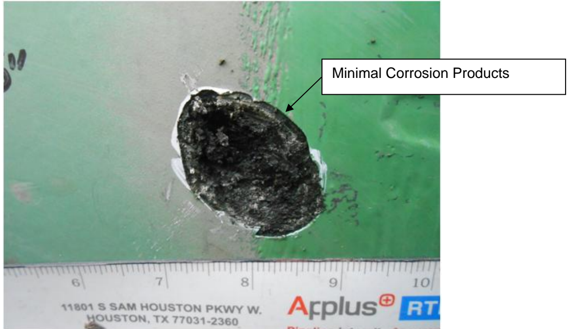
Figure 10. MP 995.95 –External Corrosion Pitting
