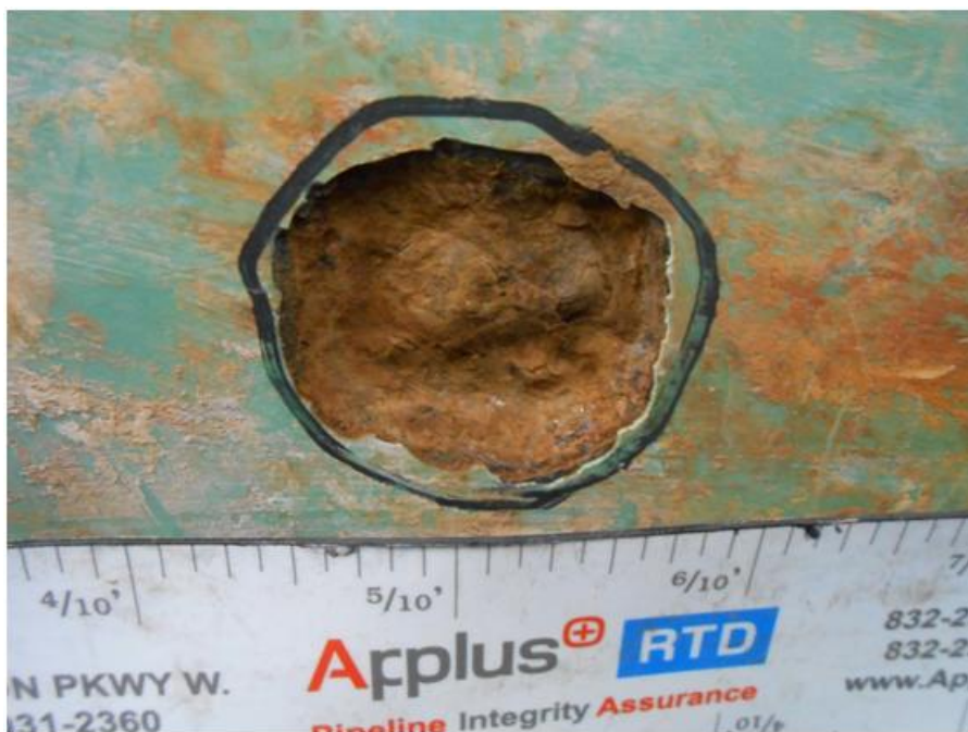
Figure 26. MP1000.32 – External Corrosion Pitting
